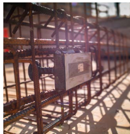
FIGURE 27 SIDE VIEW OF CONSTRUCTION SITE AT NORDBRO (LEFT). PCS® CORBEL COLUMN PART INSIDE REINFORCEMENT CAGE (RIGHT).
