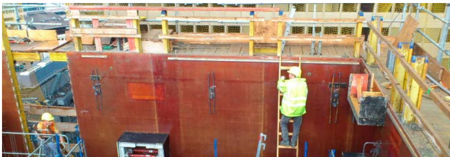
FIGURE 25 ASSEMBLY OF PCS® CORBEL COLUMN PARTS ONTO WALL MOLDS
