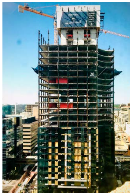
FIGURE 15 LEVEL 21 OF 300 MAIN TOWER. DELTABEAM® AND HOLLOW-CORE SLAB LAYOUT.
