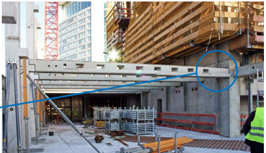
FIGURE 24 STRUCTURAL LAYOUT OF A TYPICAL FLOOR AT TAUNUSTURM, ©ED. ZÜBLIN AG (LEFT). BEAM-TO-WALL CONNECTION WITH PCS® HIDDEN CORBEL (RIGHT).
