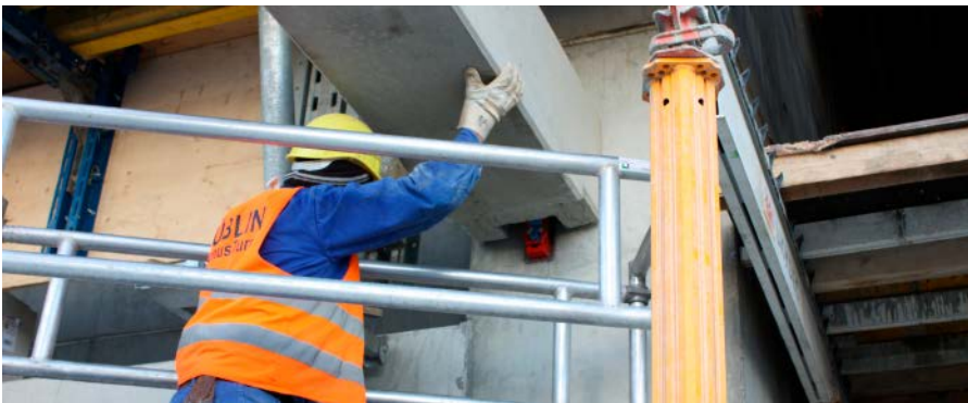
FIGURE 26 ERECTION OF THE BEAM ON PCS® CORBEL PLATE (LEFT). BOLTED PCS® CORBEL PLATE (RIGHT).
