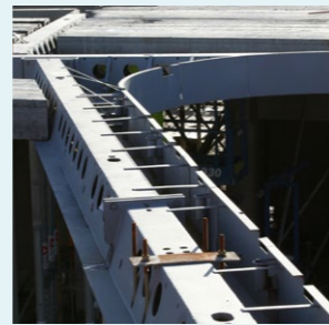
Integrated formwork for creating custom beam shapes
