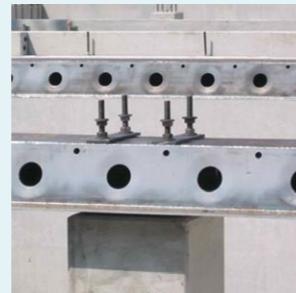
Anchor Bolts for connections on top of concrete columns
