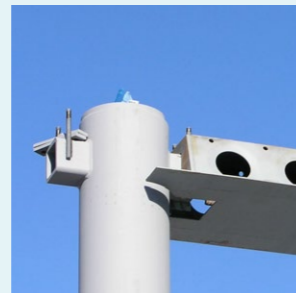
Steel column corbel connection
