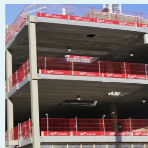
Safety rail mounting sockets for saving time and effort when installing safety rails
